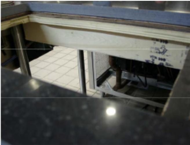
5 Support structure should be level to fully support to the Vicostone.
