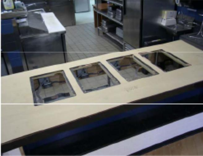
4 Support beams between cut-outs.
